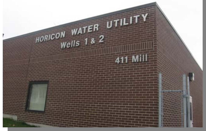
Horicon Water Utility
